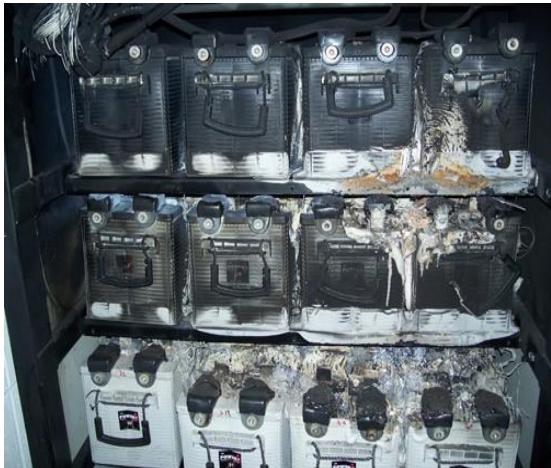
Container Destruction due to Thermal Runaway
