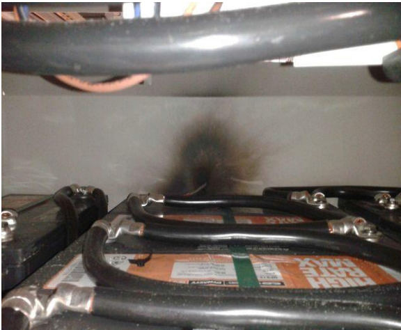
Explosion due to Thermal Runaway
